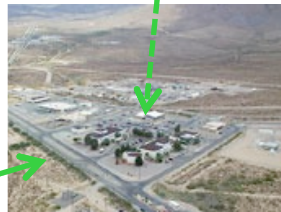
White Sands Ground Terminal, NM
